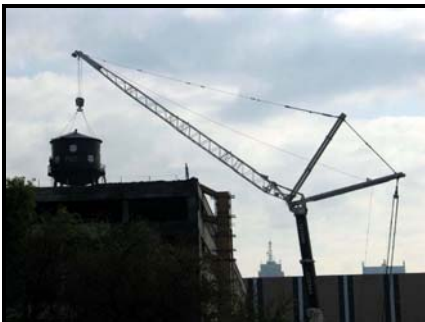
Water Tower Removal
