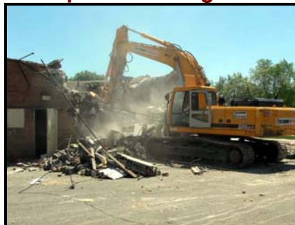
Complete Building Demo
