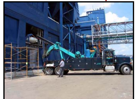
Removal in Confined Spaces
